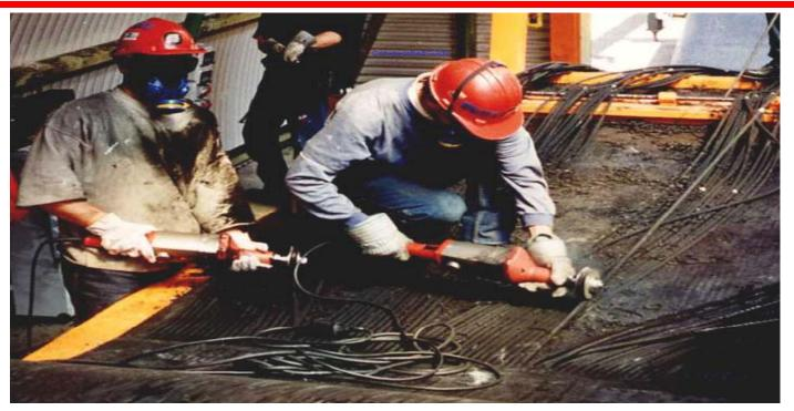
The top and bottom sides and the ends of the separated steel cords will be brushed with a grooved wire brush.
