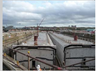
New Submersible sections for the Tunnel
