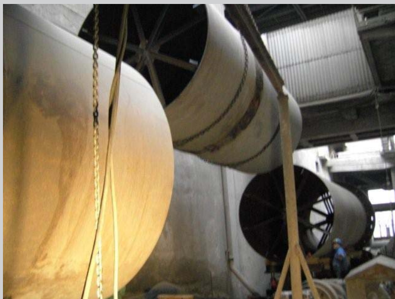
Disassembly kiln shell
