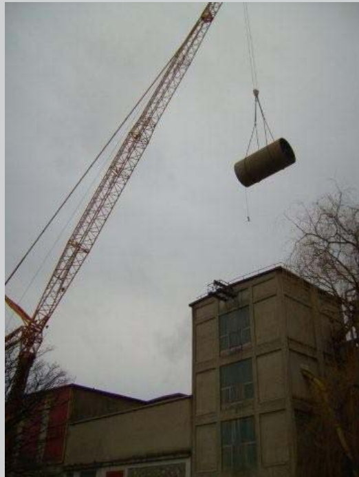
Lifting kiln shell out of the building
