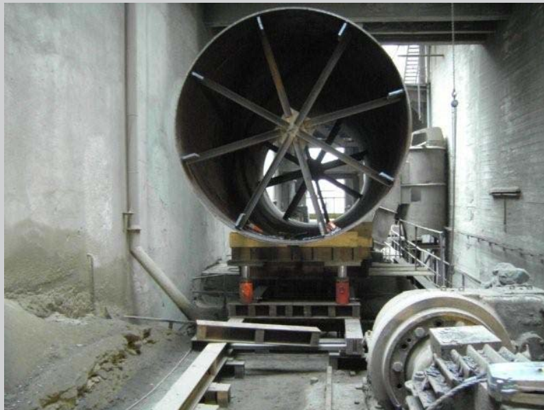
Temporary support at the disassembly kiln shell
