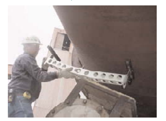
Carrying Roller Adjustment
