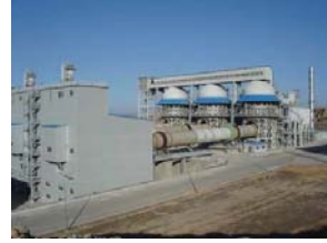
Lime Plant Maintenance and Processes
