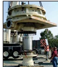
Bottom Shell Lowered onto Eccentric
