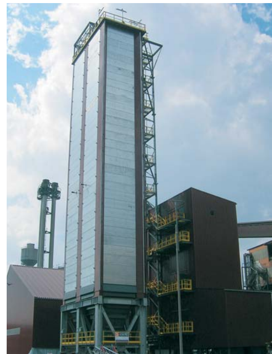
Austria, plastic pellets ● poor flow characteristics, 2 cells of 800m 3 (extension to 5 cells in preparation)
