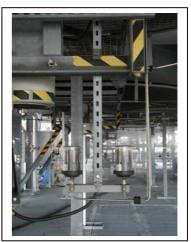
Lubrication of mechanical equipment in a chemical plant needing EX approved devices
