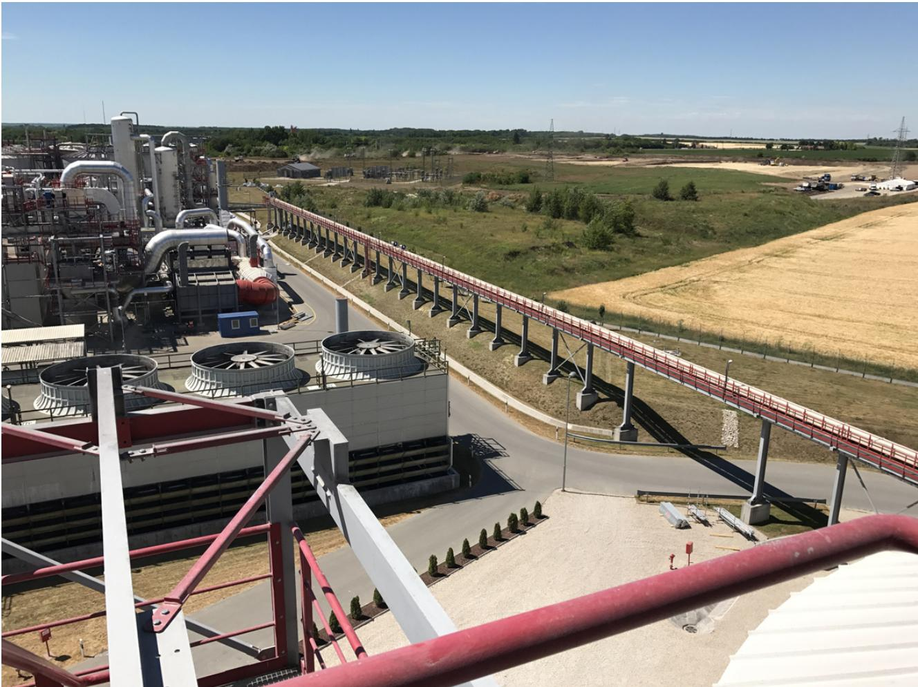
**Powerful air cushion supports the conveyor belt without the need for rollers**
