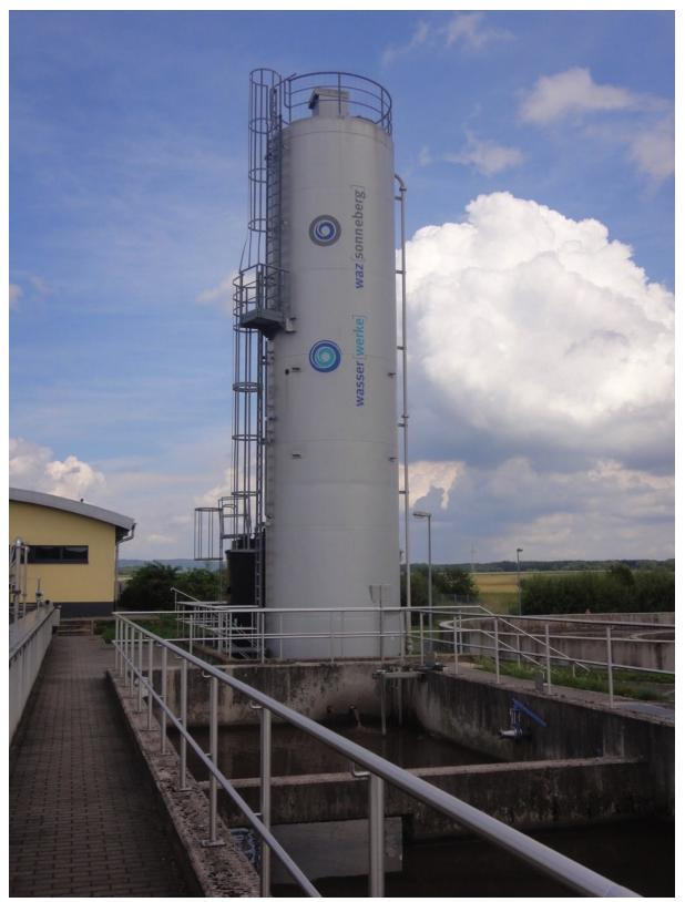
Lime hydrate must be added to the wastewater due to the very soft nature of the water in Sonneberg. (Picture: ©GKD)
