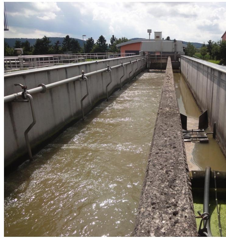
In the sand trap any sand in the material is released, washed and dewatered, allowing it to be used as backfill material in ditch and trench digging operations. (Picture: ©GKD)
