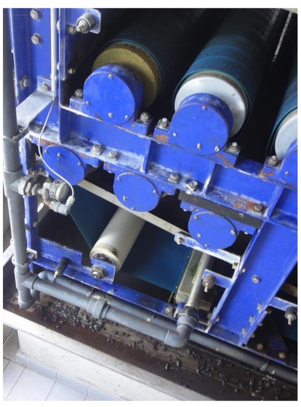
In the pressing area the sludge passes through eleven rollers between the upper and lower belt with belt pressure of 8 bar. (Picture: ©GKD)
