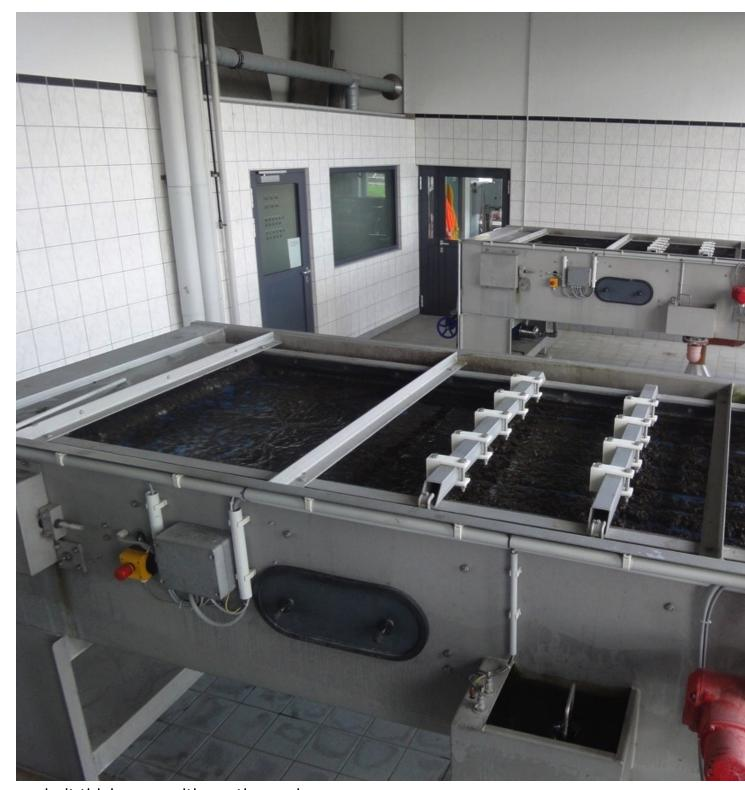
wo belt thickeners with continuously circulating Type 5060 GKD filter belts increase the solids content of the surplus sludge from 0.75% TS to around 5% TS through the addition of flocculant. (Picture: ©GKD)
