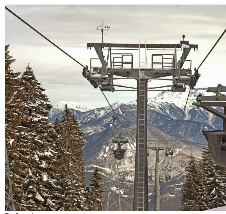
The Doppelmayr ropeway at Ceratteppe transports the ore into the valley over a distance of 4.5km across steep, wooded terrain. (Picture: Doppelmayr)
