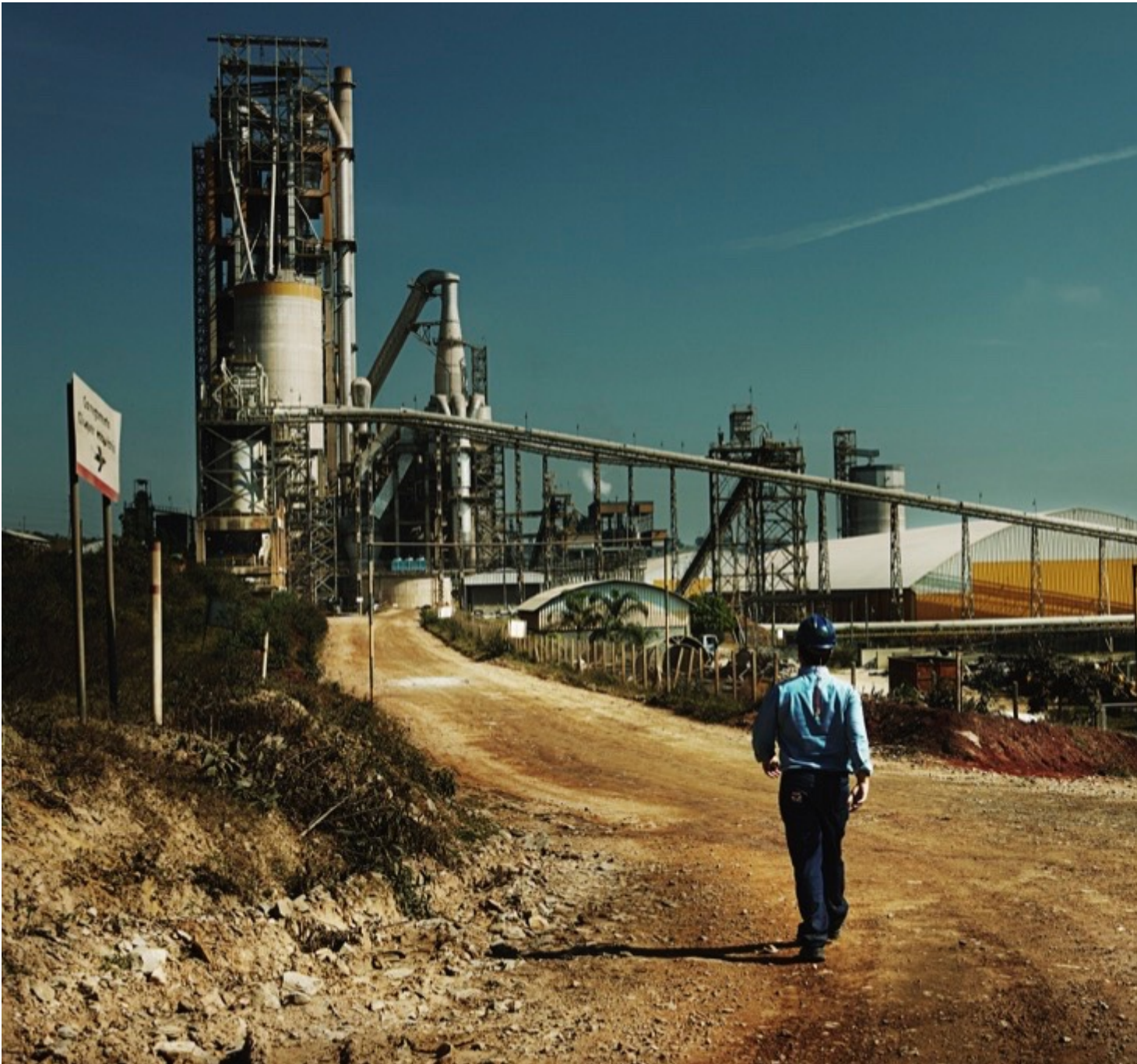
Example picture of a cement plant in Brazil. (Picture: FLSmidth)
