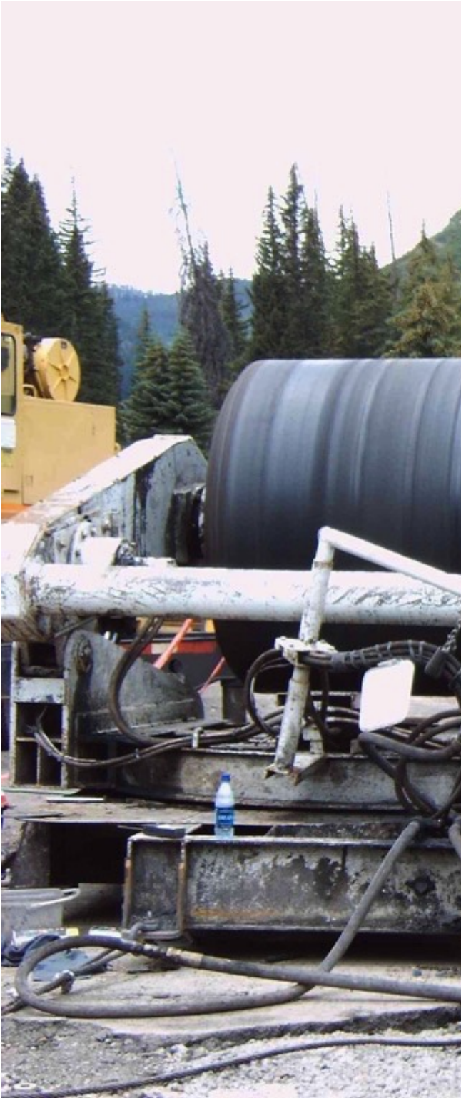
Fig. 10: Pulling the new pipe conveyor belt into the conveyor structure.
