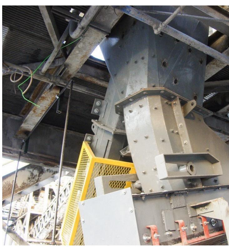
The rear chute wall in this image is bolted onto side flanges, allowing safer access. (© Martin 2020)
