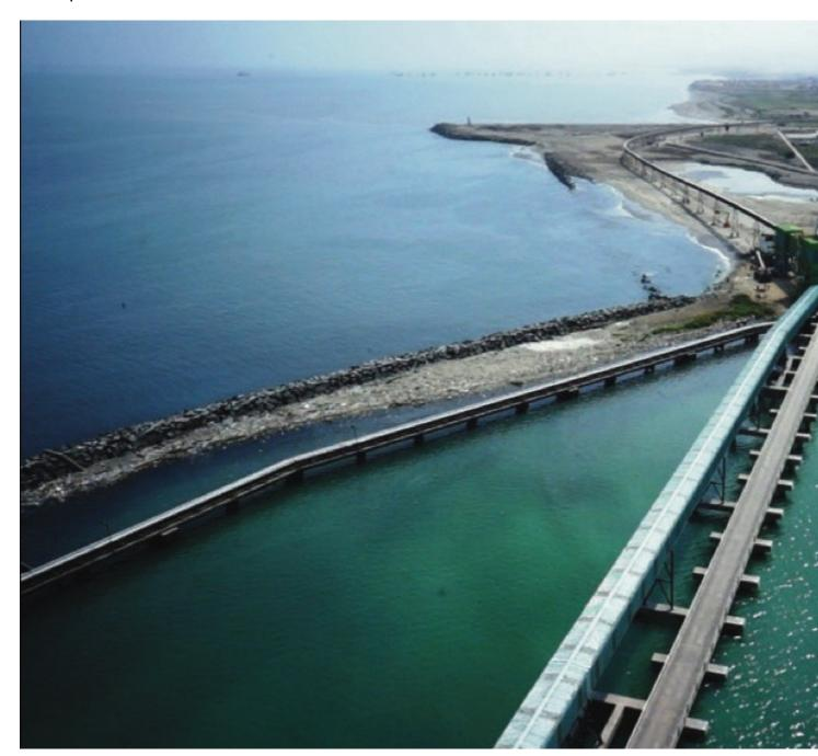
View from the pier: the last section of the pipe conveyor runs along the sea to the transfer tower.
