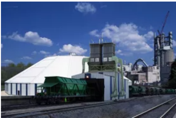
Hopper bottom railcar discharge to circular storage.
