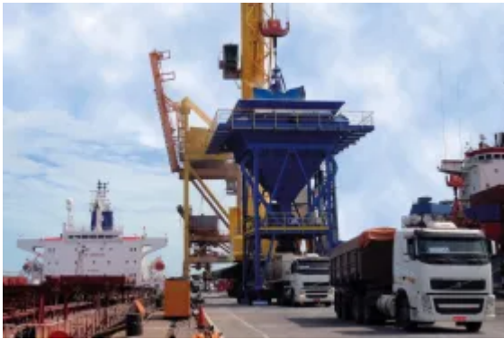
Dust controlled tyre mounted Eco-Hopper ship discharge to tipping truck.
