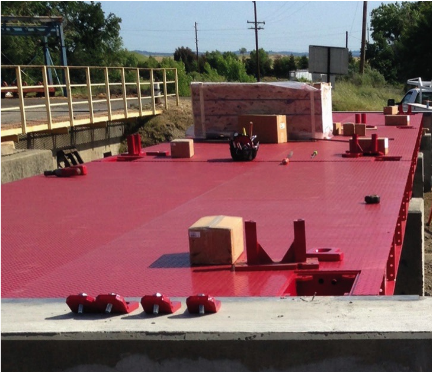
Belt scale during erection.
