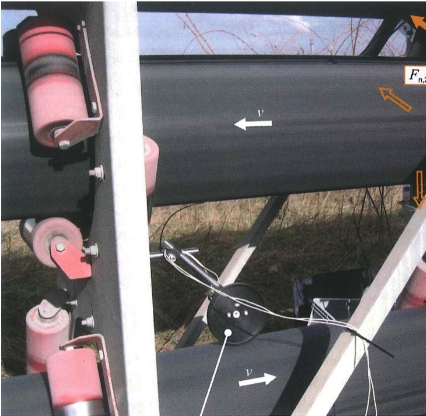
Fig. 9: Pipe conveyor in Portland-Zementwerk Wittekind of Hugo Miebach Söhne, used by Hötte for his field measurements, Institute of Transport and Automation Technology (ITA) at Leibniz University of Hannover [14]. (Picture: © S. Hötte, Leibniz University Hannover [14])
