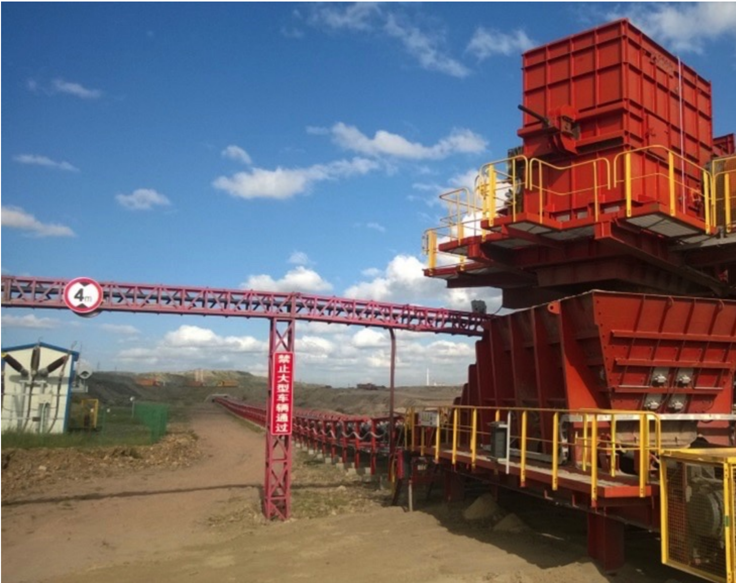
Conveyor transfer station at Zhahanaoer.
