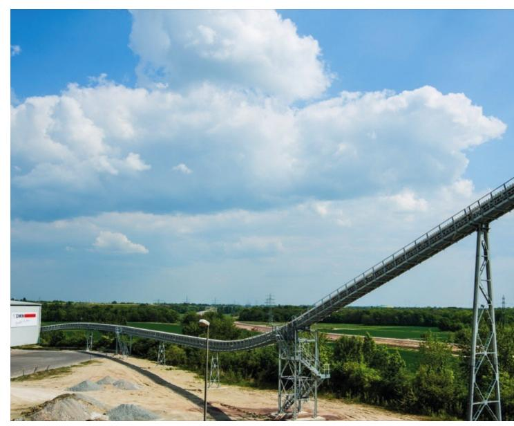
The fully closed pipe conveyor system makes elevated bulk material transport safer, more environmentally friendly and energy efficient. (Pictures: ©Beumer Group GmbH & Co. KG)
