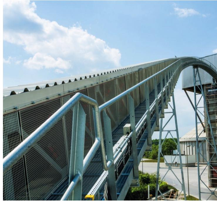
The discharge station shown is at a height of 26 m were the material is transferred onto the feeding system for the main burner.
