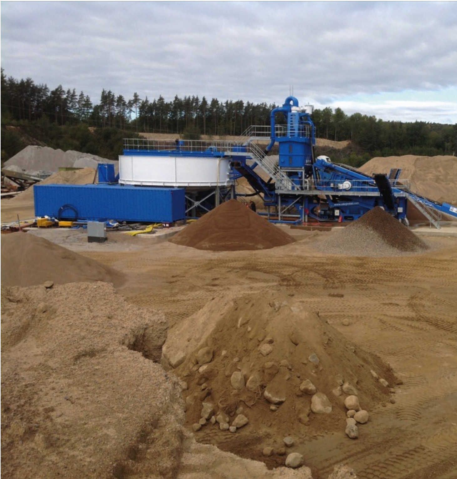
The new sand and gravel washing plant of Bröderna Björklund Grus in Olofström. (Picture: ©CDE Global)
