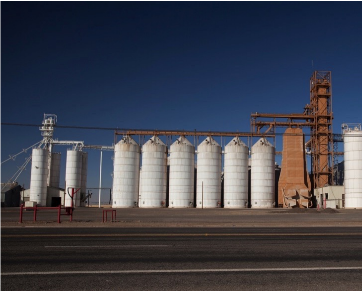
Fig. 1: For many applications reliable flow from a silo is a pre-condition for an efficient and economic downstream process chain.
