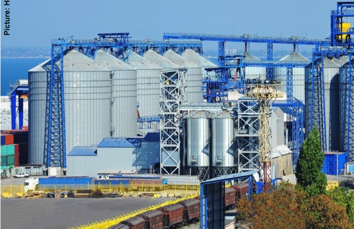
Fig. 1: The dynamic pressure acting on on the silo wall during discharge is directly related to pattern of material flow in silos.
