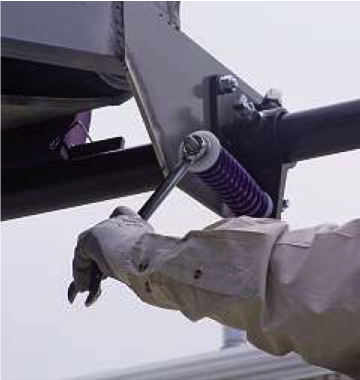
Fig. 4: Fixing a problem with carryback may be as simple as adjusting the tension on cleaners.
