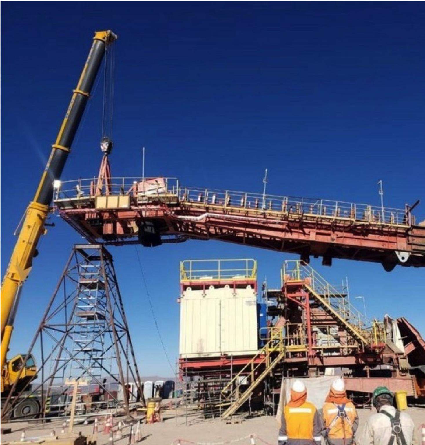
Installation of the boom into the superstructure of the TAKRAF BWR 7100 at the mine in Chile. (Picture: ©TAKRAF)
