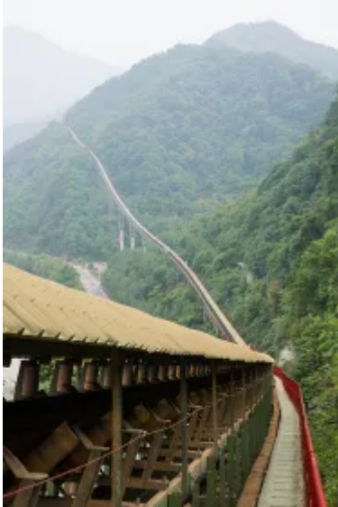
Sichuan project: The troughed belt conveyor runs through rough terrain and over instable ground.
