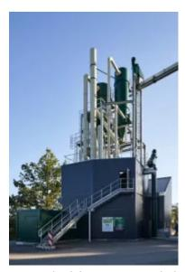
By switching to wood dust, the plant operator has ensured virtually carbon-neutral production for the asphalt while also cutting costs by 20%.
