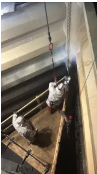
REMAPUR-75 applied in multi-chamber silo
