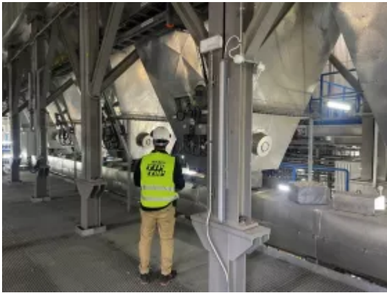
Maintenance Inspection in a Middle Eastern process plant
