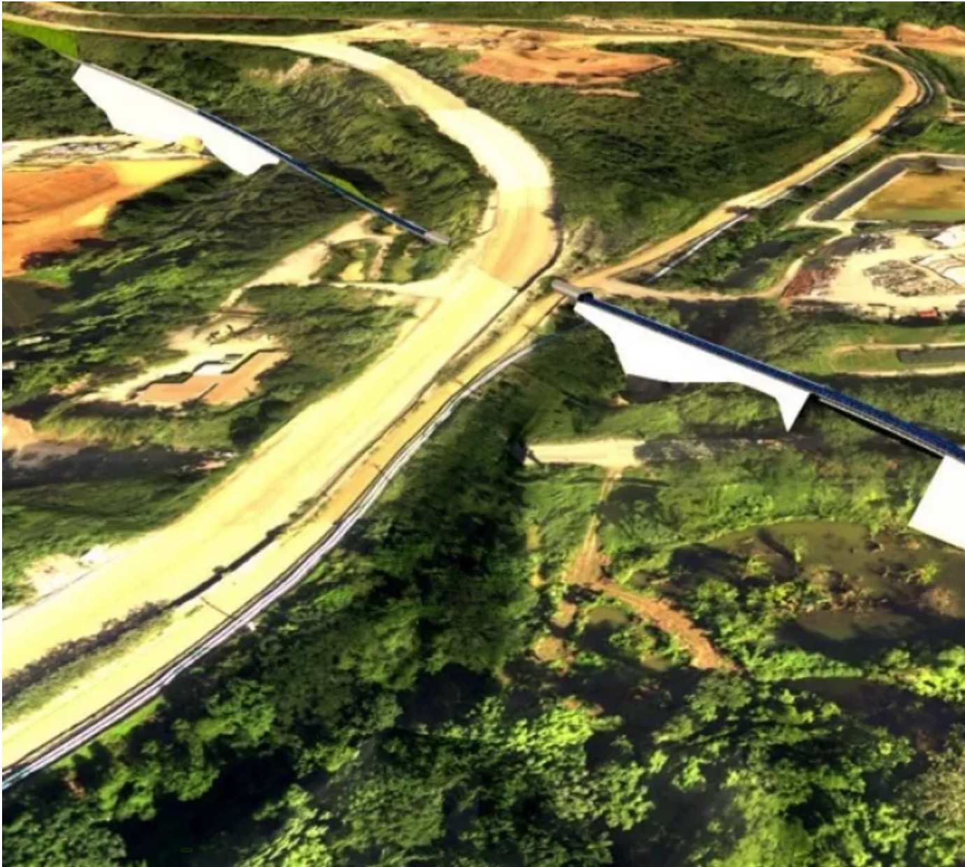
A 3D model of terrain and conveyor: the advantages of earthworks (cut & fill) or steel
