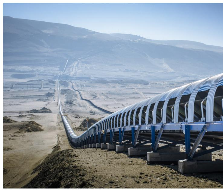
thyssenkrupp belt conveyor systems are individually planned and constructed to ensure the best possible solution for every material, every climate zone and, every topography. This downhill conveying system installed in Peru transports 4,500 tons of crushed iron ore from mine to the port.
