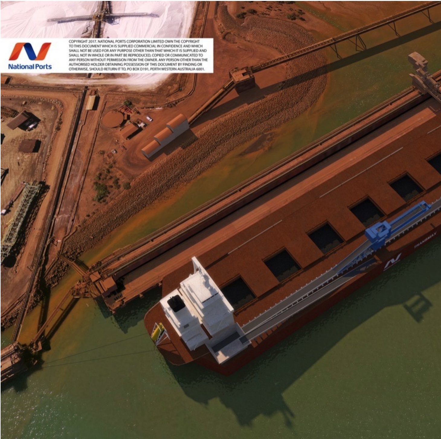
Loading a Transmax at Port Hedland, Australia (graphic representation).
