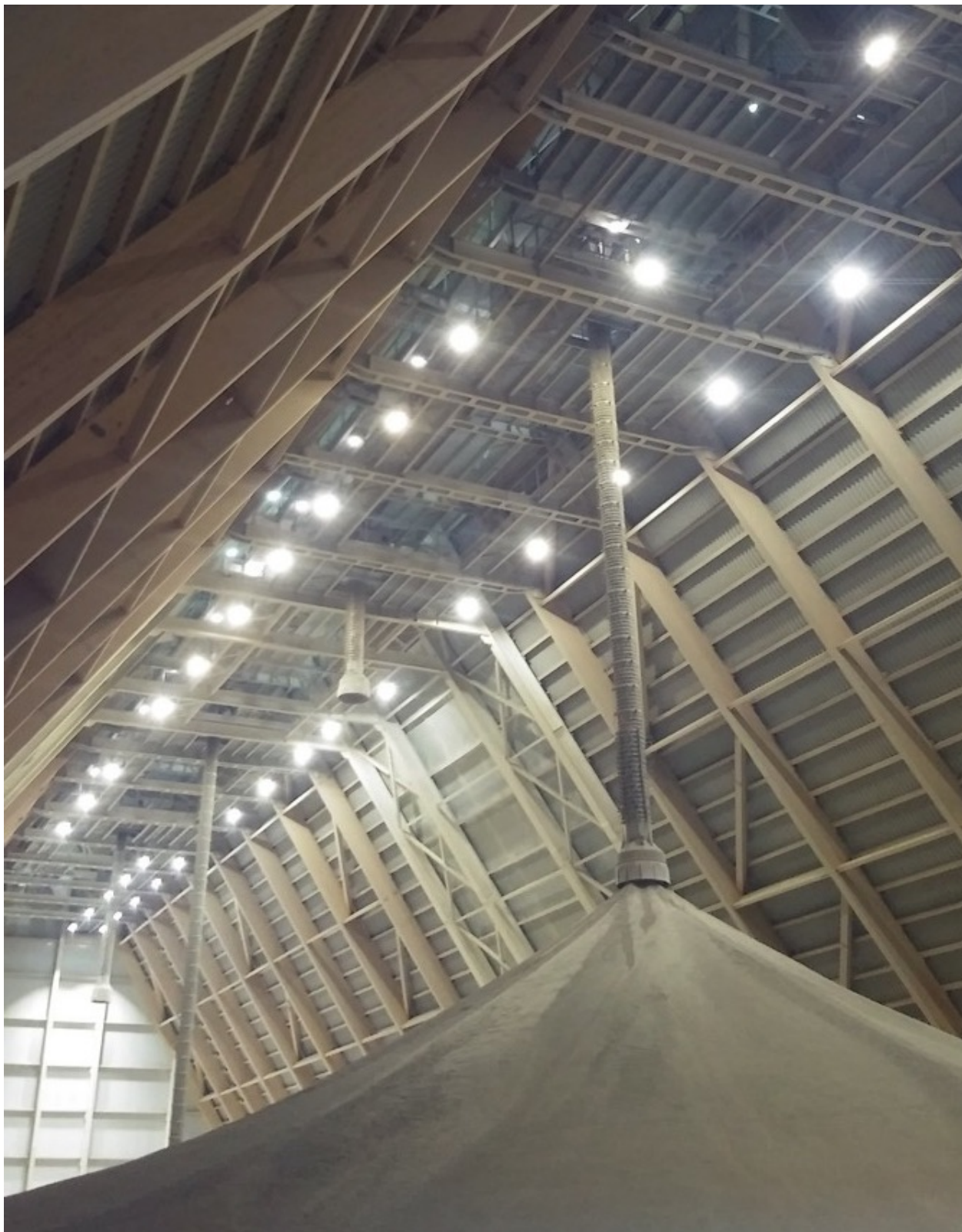
Unloading of phosphate into a warehouse.
