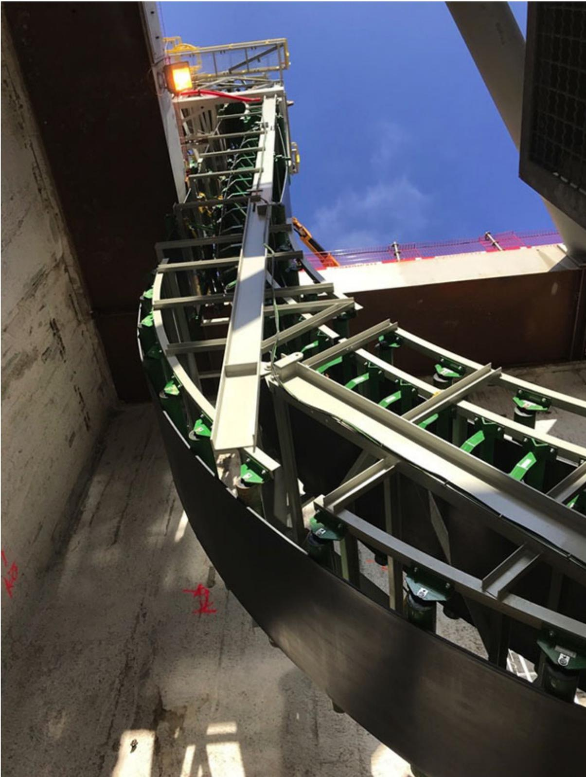
DSI GPS is able to elevate material economically, at high volumetric rates in limited vault space.
