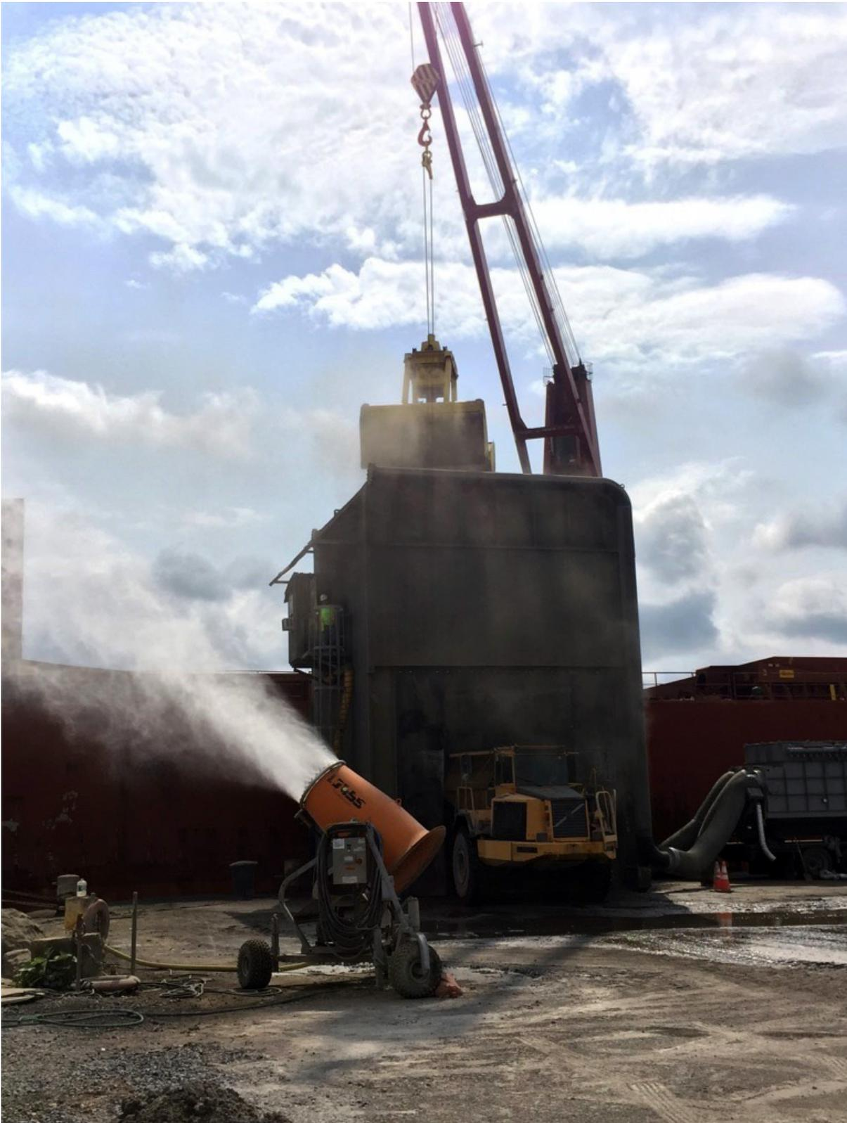
The compact size of the DustBoss allows easy positioning, and it can run continuously unattended.
