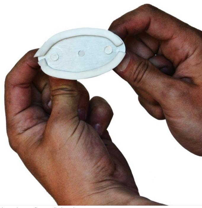
Adhesive strips are first applied on the perimeter of the mounting base.
