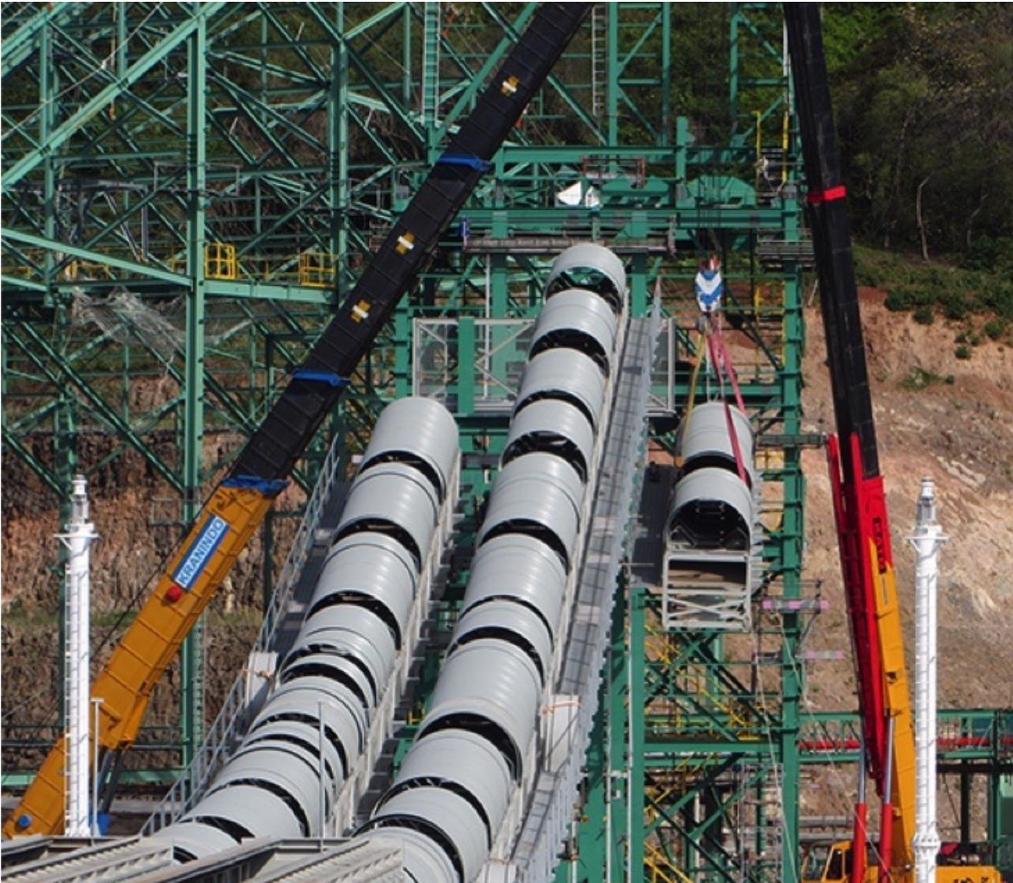
Siwertell's Modular Belt Conveyor System comprises precision-engineered, lightweight, prefabricated frame modules, which can be designed horizontally, or to various inclines.
