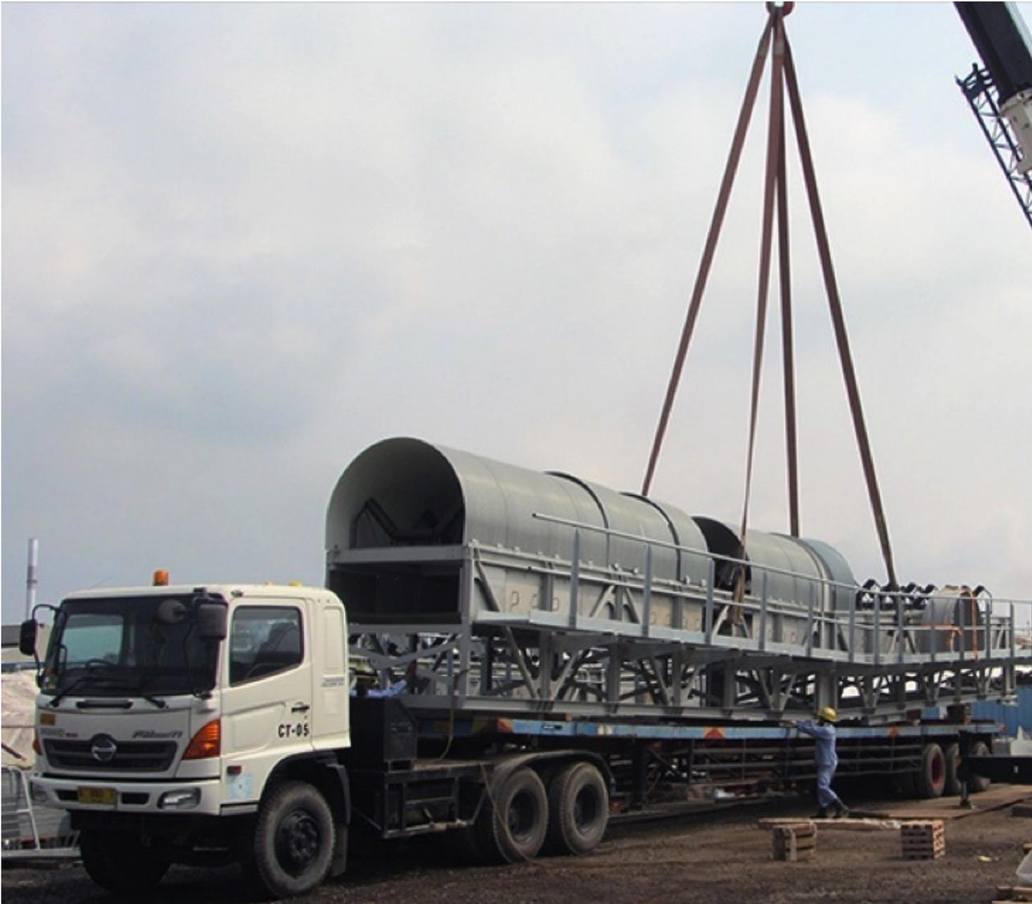
With the help of an assisting crane, the pre-assembly phase of the installation, involving the assembly of the 18 m prefabricated module sections, was completed in the space of only two days.
