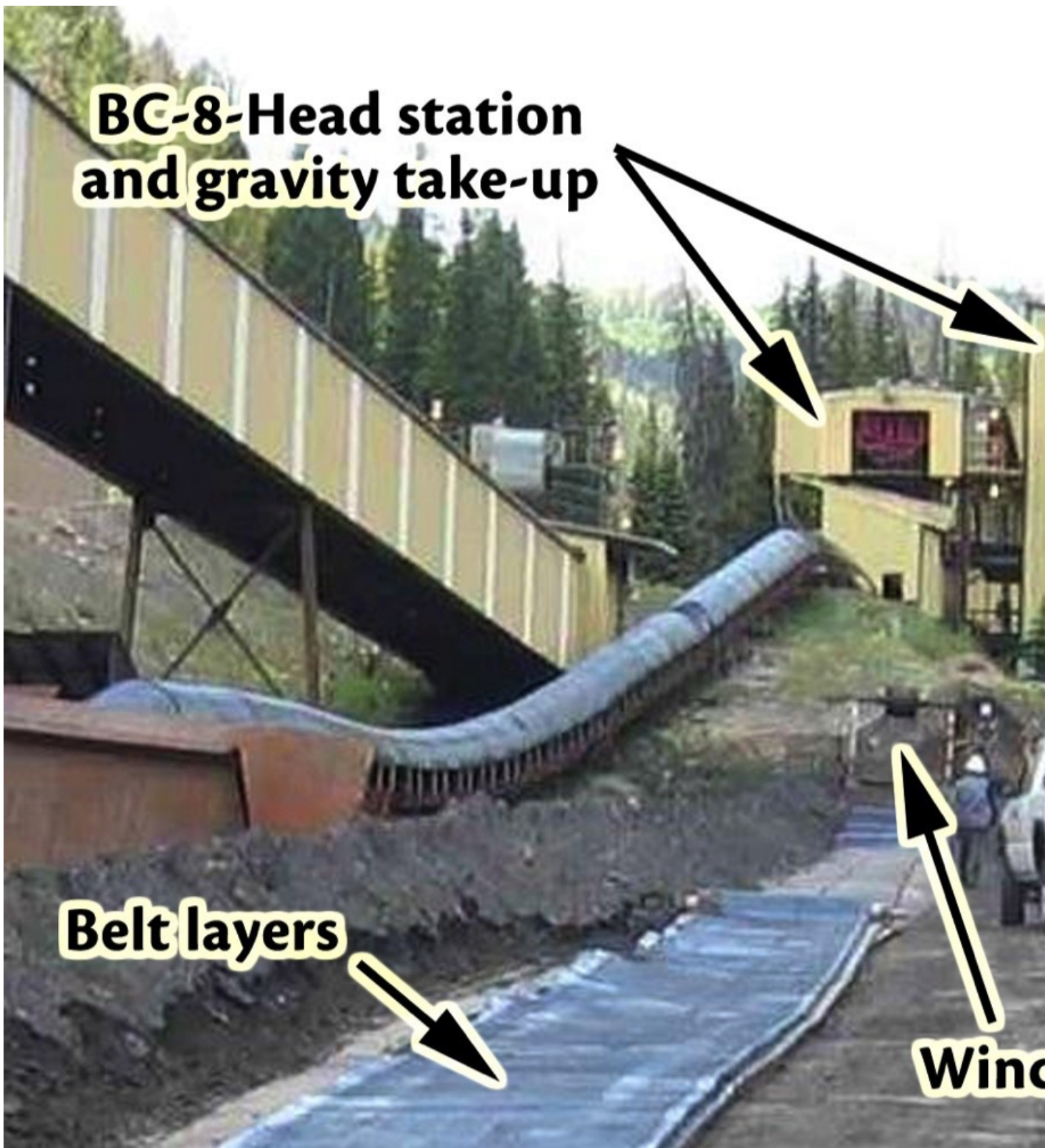
Fig. 7: Reeving of the belt with a winch.
