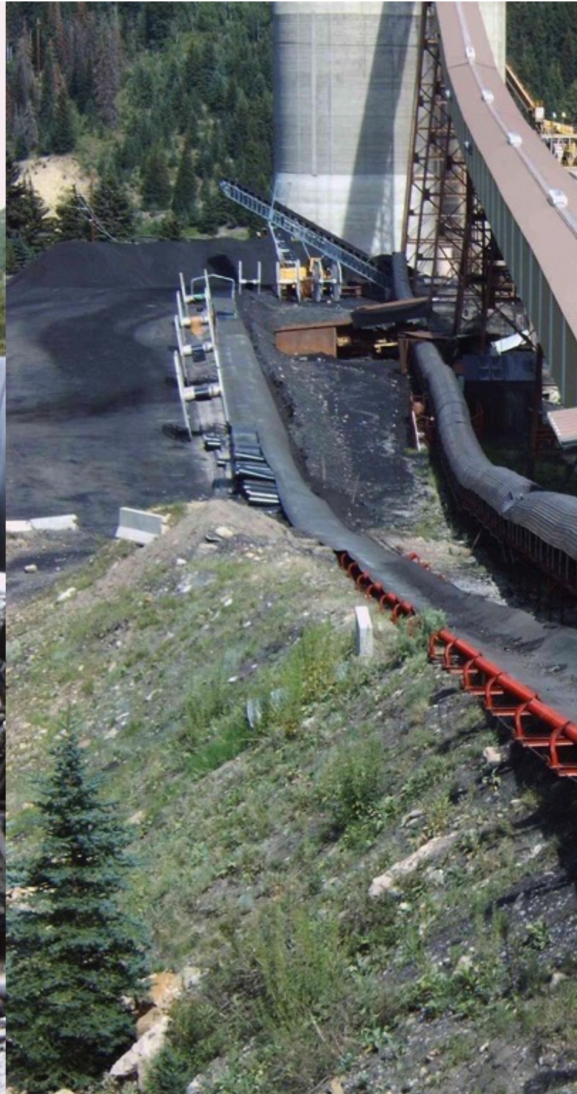
Fig. 11: A temporary conveyor was installed to reduce friction.
