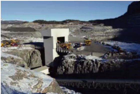
Direct feed semi-mobile crushing plant at Norsk Stein AS, Norway.
