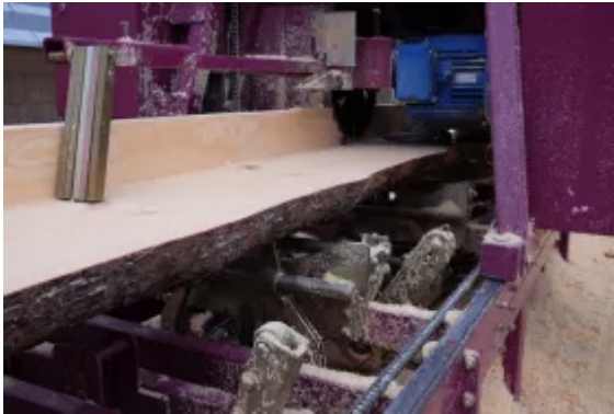
Highest priority for explosion protection at wood-processing plants
