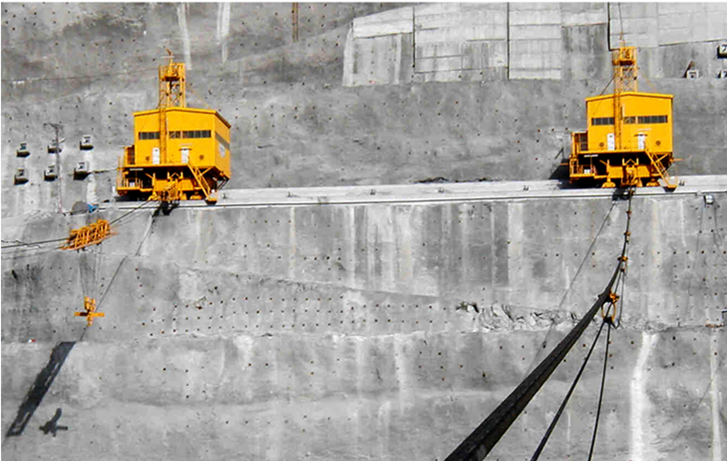
Fig. 2: Thyssenkrupp cable cranes for dam construction.
