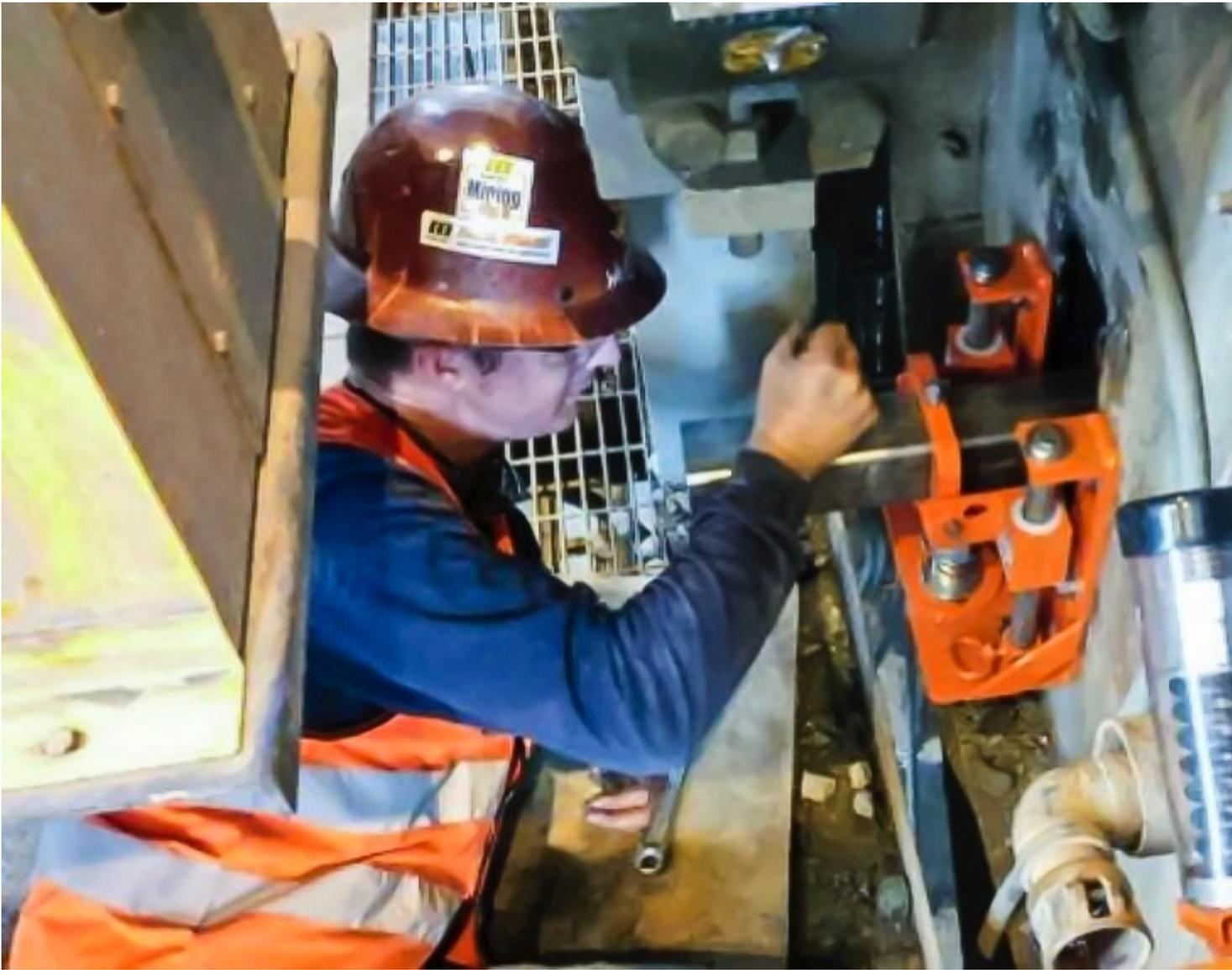
Martin Engineering replaced existing primary cleaners at sixteen discharge points, fitting them with low-adhesion urethane blades.
