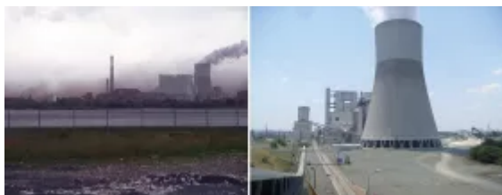
Fig. 1: Old (left) and new (right) part of the Maritza East-1 power plant. (Pictures: Contitech, Takraf)
