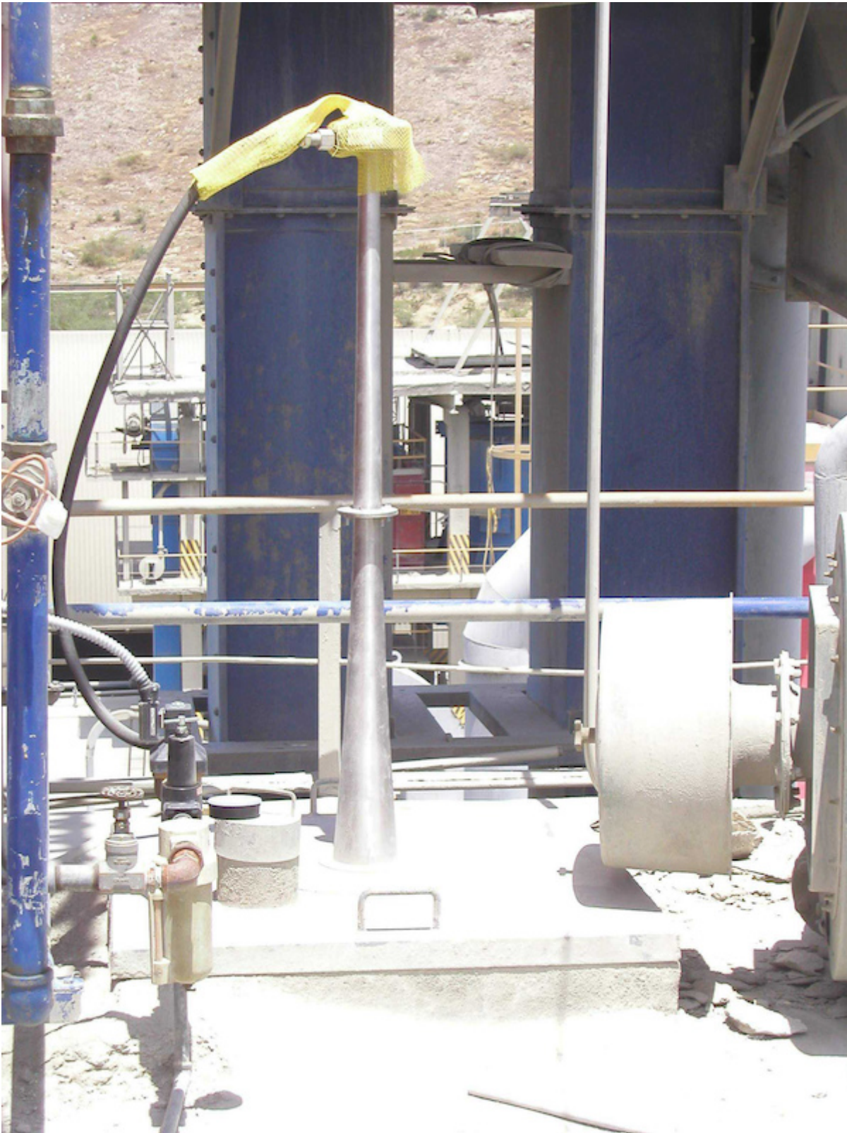
Typical installation of an acoustic cleaner on top of a silo.
