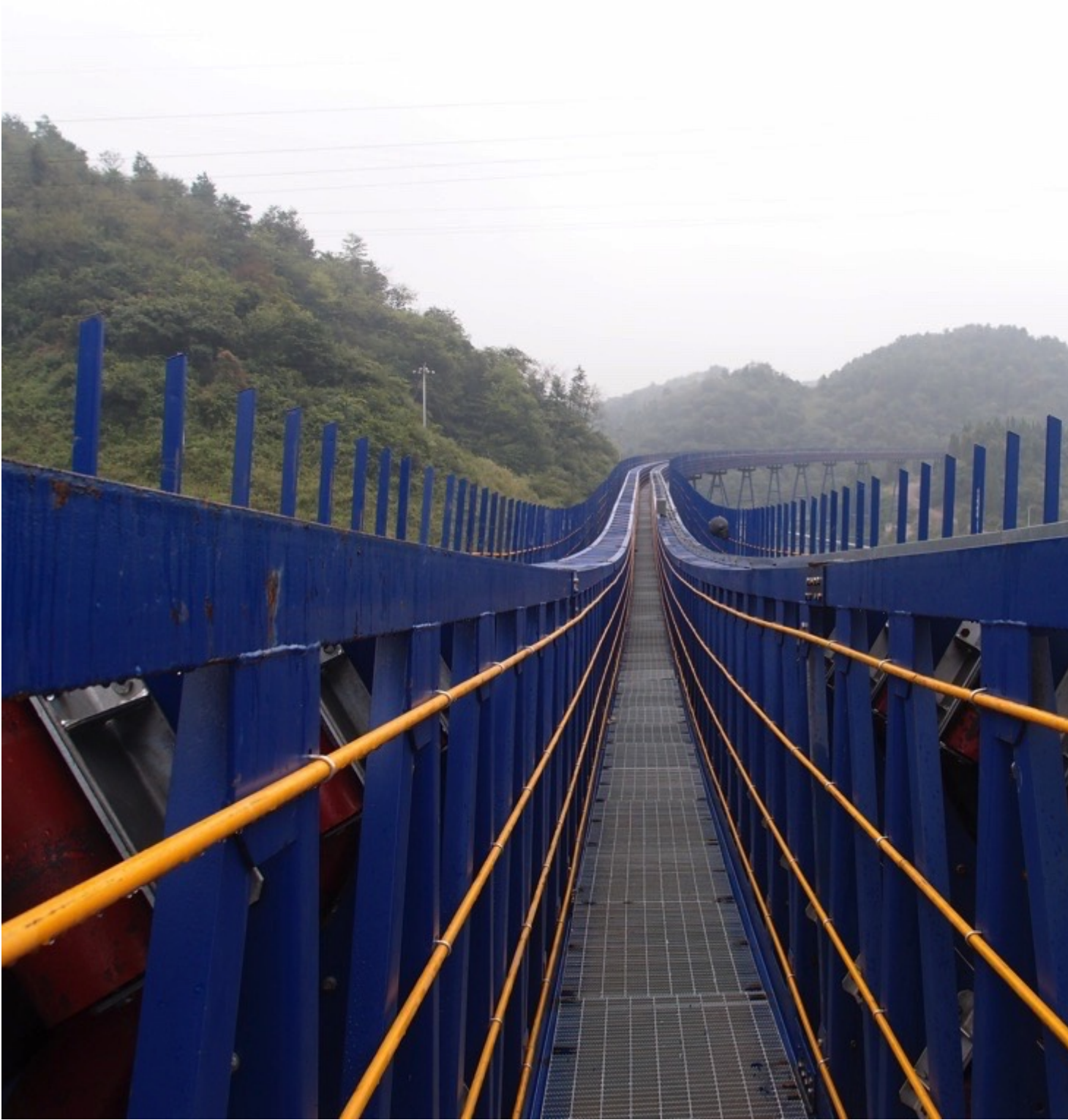
Fig. 6: Parallel 6.2 km Kailin pipe conveyors, LRR pipe belt along with Conventional pipe belt.
