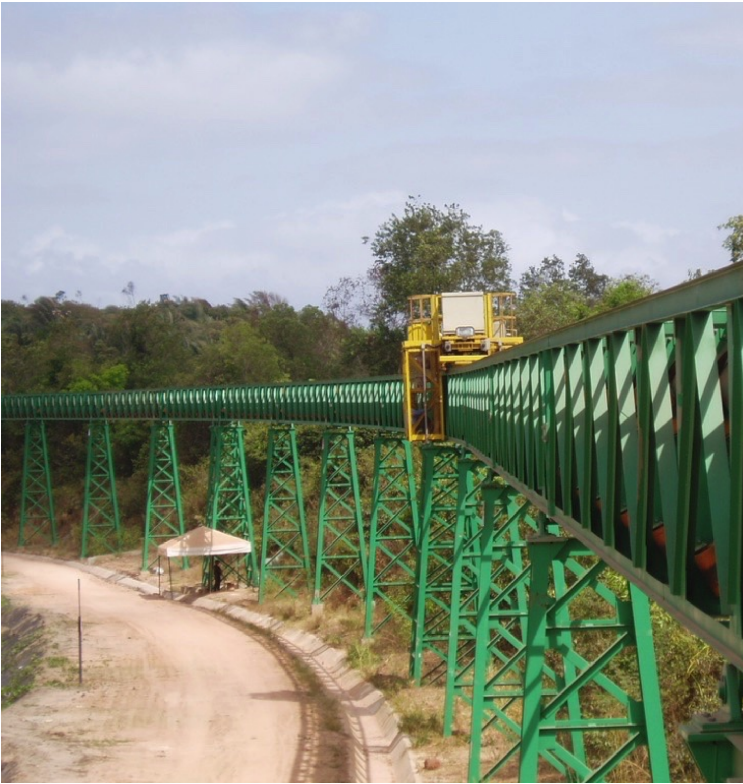
Fig. 1: The 4.3 km long Brazil Itaqui PC1 pipe conveyor is equipped with a ST1400 Super Low Rolling Resistance pipe belt. (Pictures: © Conveyor Dynamics, Inc.)
