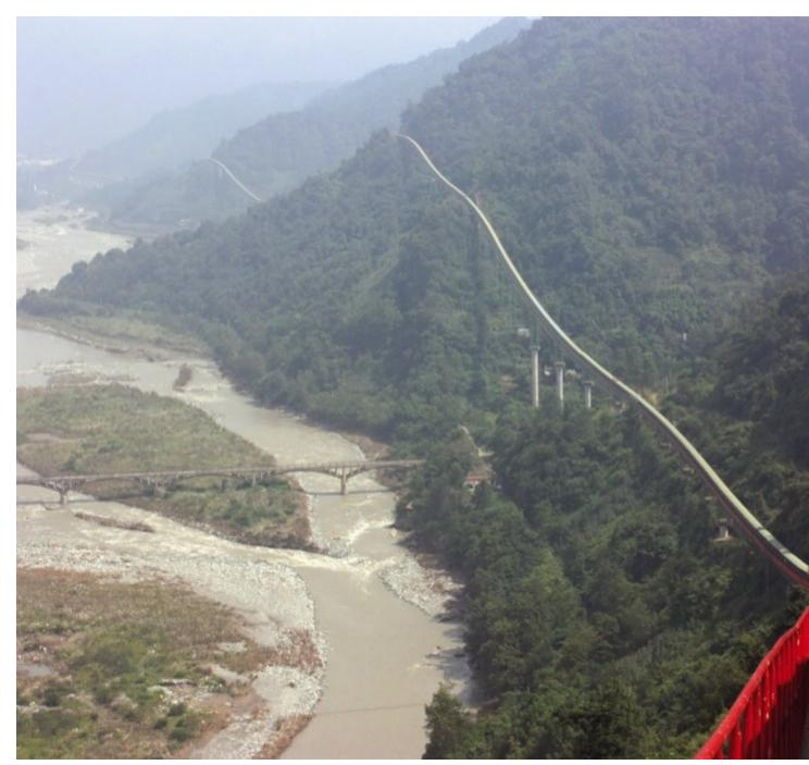
Belt conveyors: rapid and efficient transport of bulk material from the quarry to the destination as well as through rough terrain. (Pictures: © Beumer Group)
