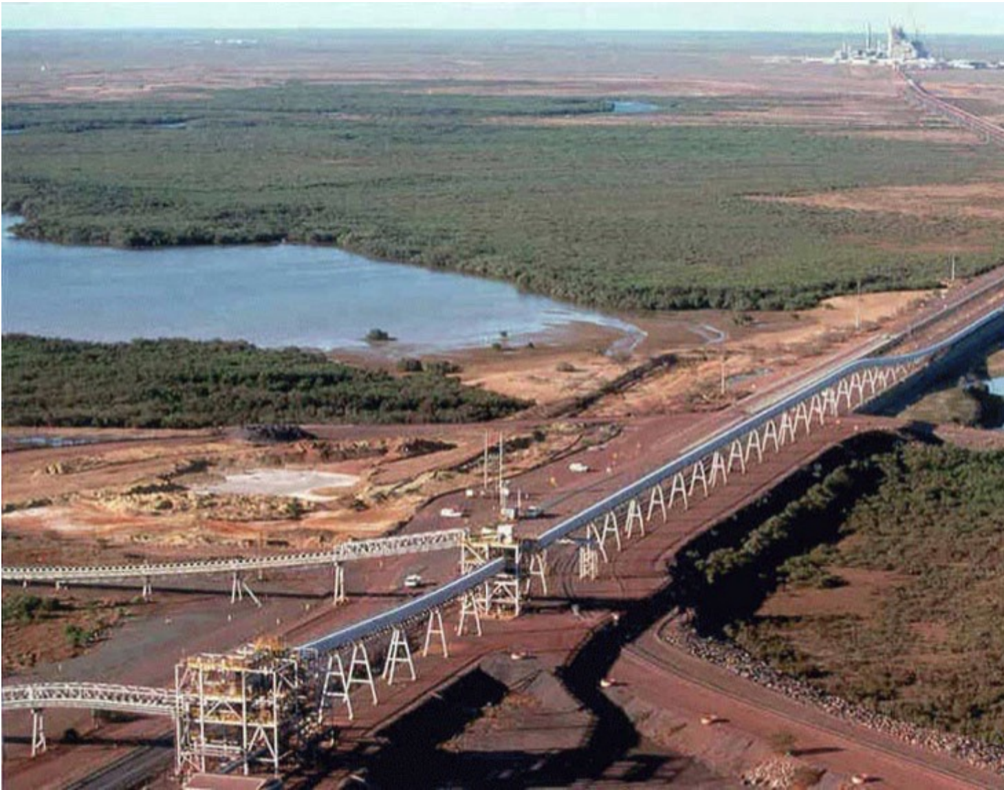
Fig. 1: Conventional troughing overland conveyor, Boodarie, Western Australia. (Picture: Bechtel Corporation)
