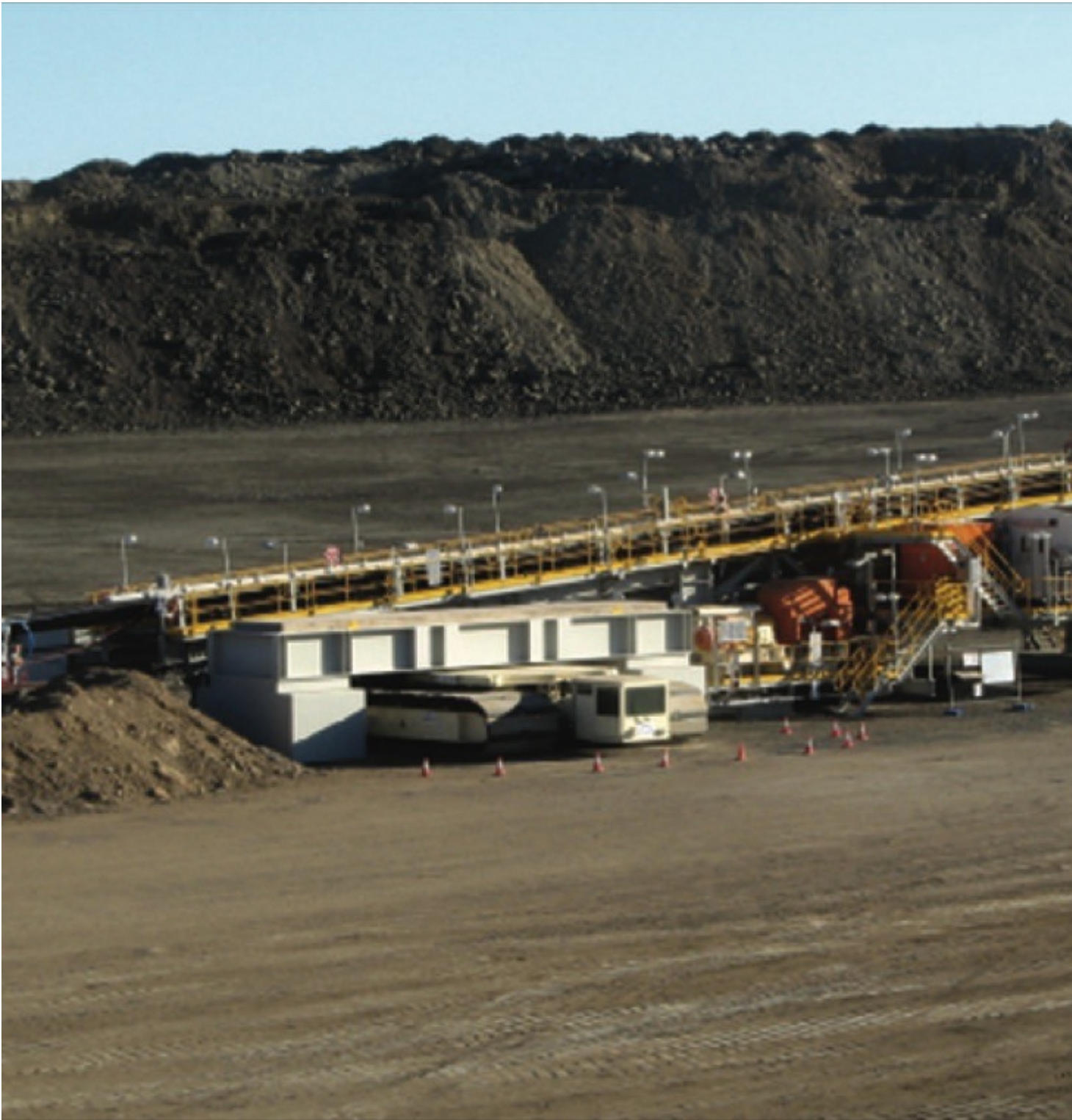
Fig. 9: Mobile transport crawler under relocatable drive head restraining mass. (Picture: Sinclair Knight Merz)
