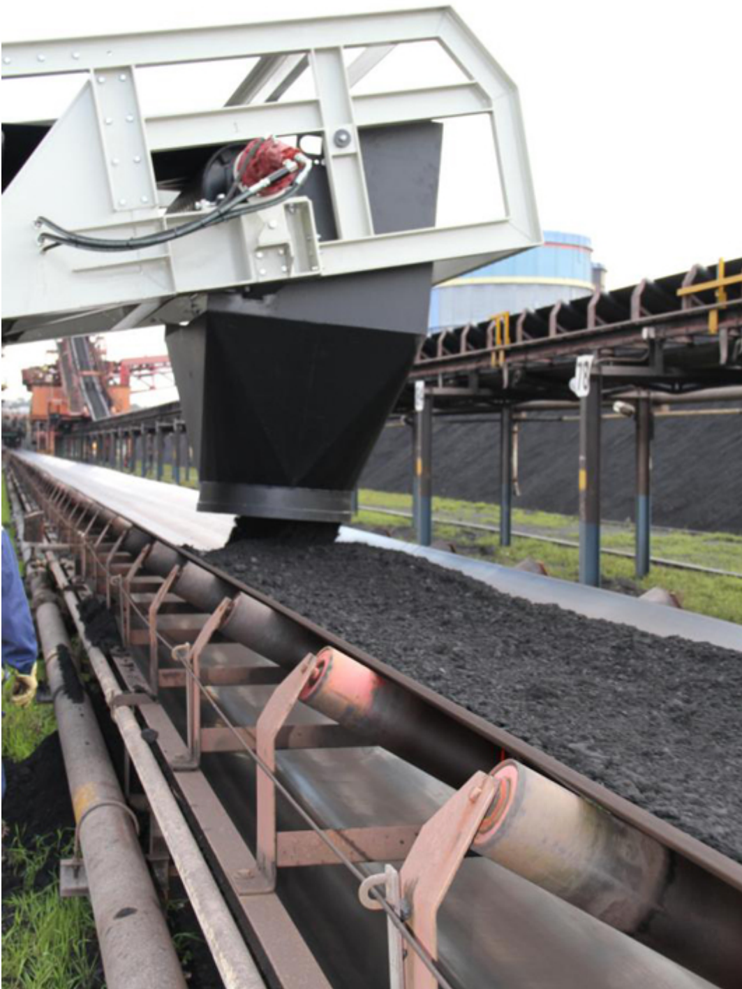
Fig. 4: The material is directly transferred on an overland conveyor system.
