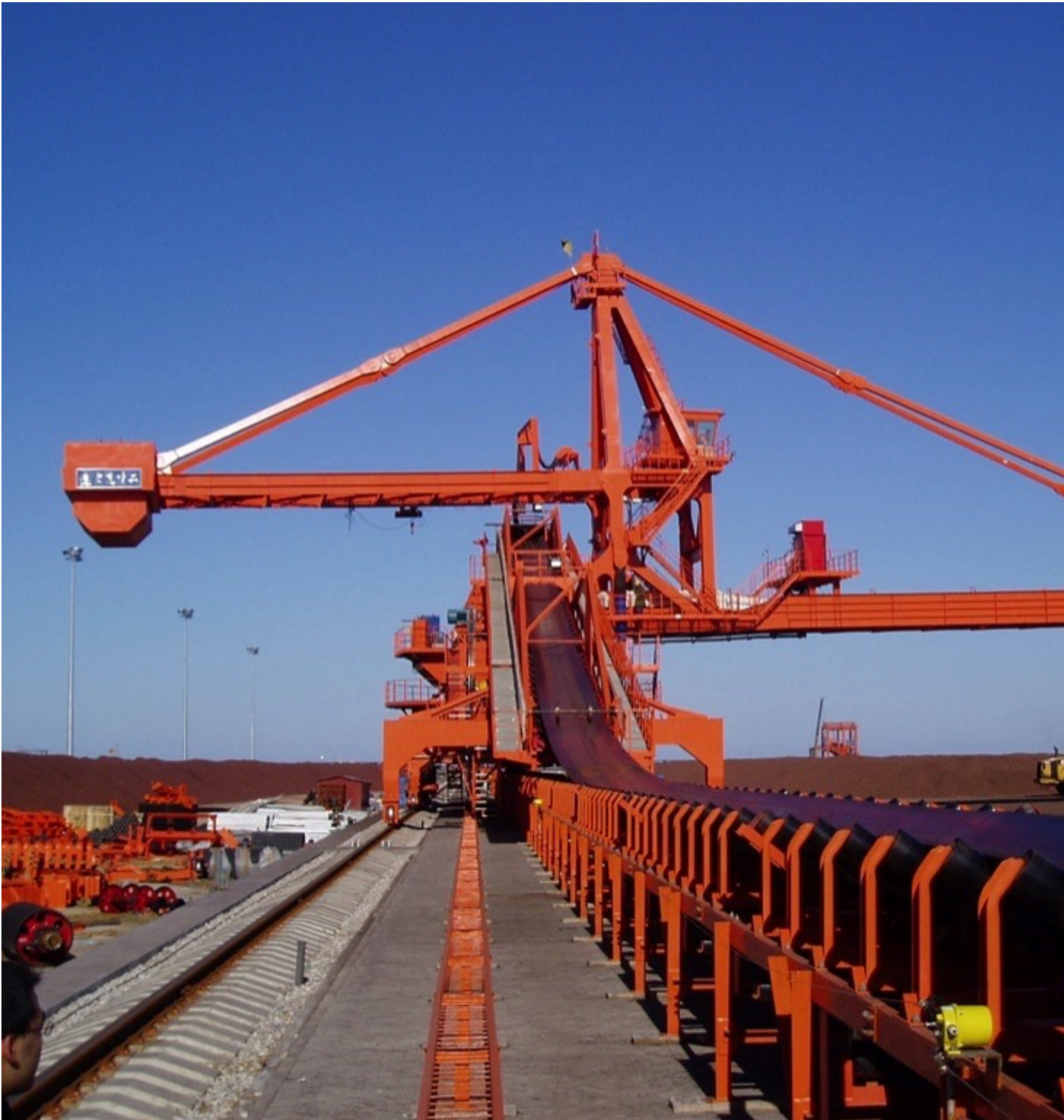
Fig. 7: Stacker reclaimer with slewable and luffable boom. (Picture: © DHI DCW Group)
