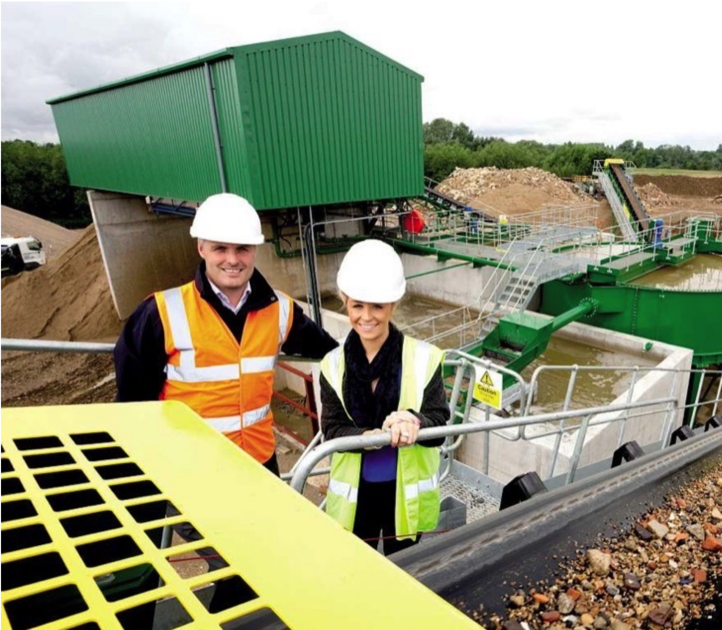
Fig. 1: The waste water treatment plant first involves the thickener, which receives waste water from the Evowash. (Pictures: CDE Global Ltd.)
