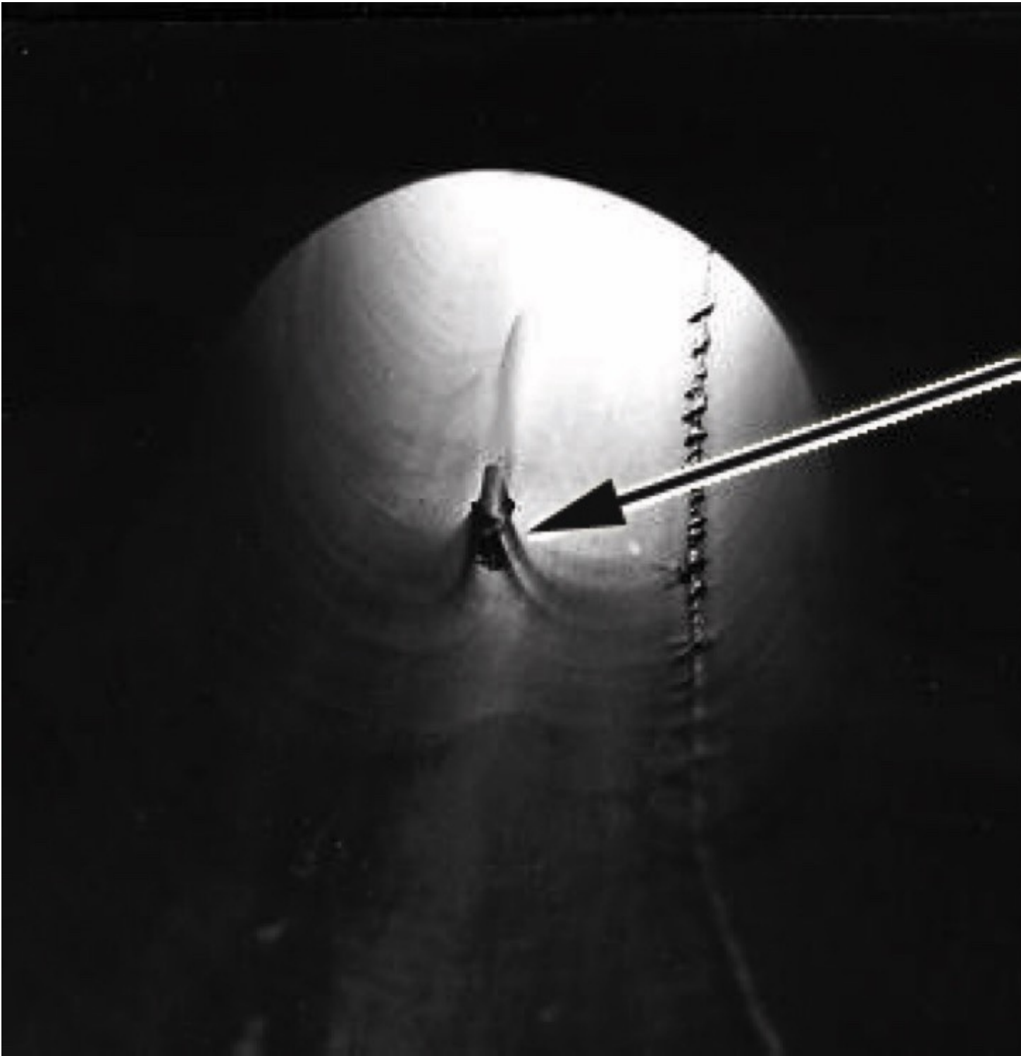
Fig. 3: Photograph of a typical pneumatic conveying line puncture (viewed from inside the pipe, and from the direction of flow)
